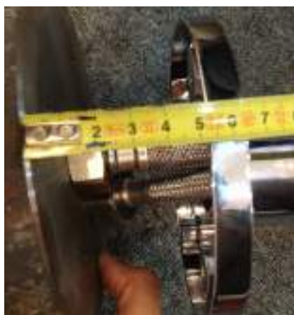
Note: Flexible hoses stick out by 50mm
